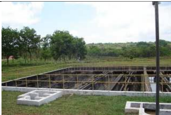
Figura 1: Reator UASB
